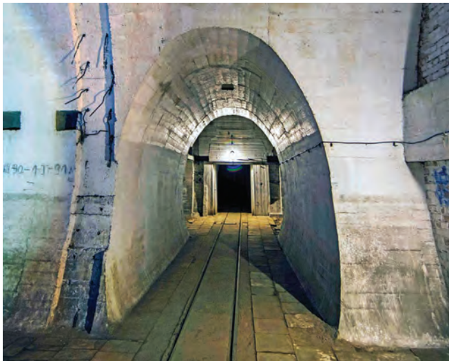
In the first part of the MRU system we visited, near to the bottom of our entrance shaft
